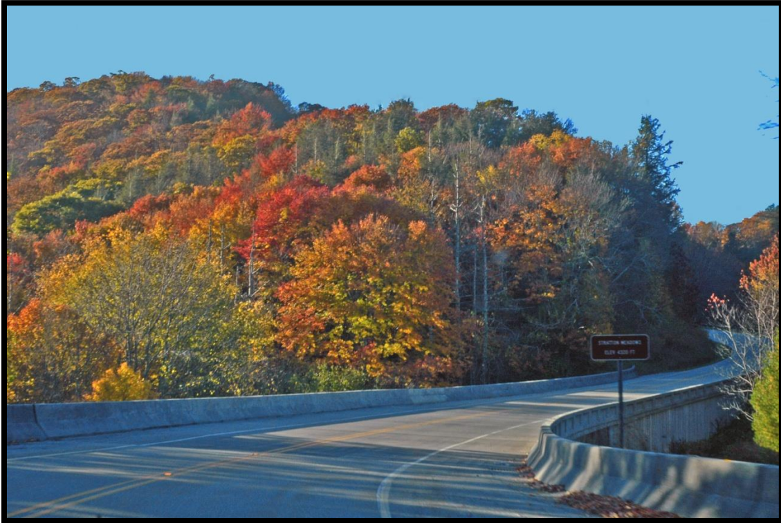
The Skyway is a two-lane road following the mountain ridges where possible, with concrete bridges where necessary, such as this one spanning Stratton Meadows.
